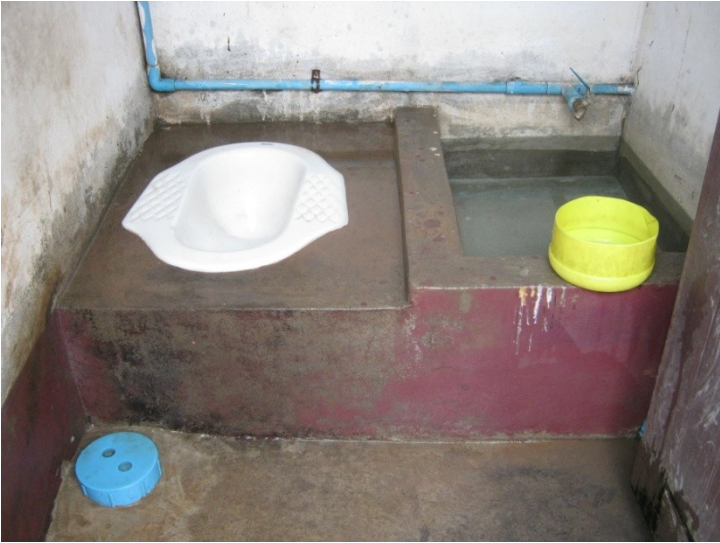
Newly constructed toilet, Lao PDR
