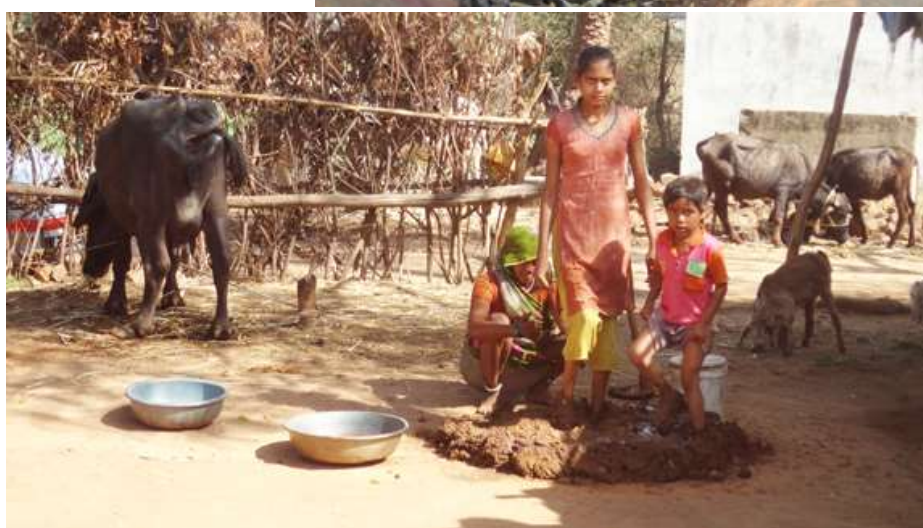
Mixing water, dung and mud for plastering the floor
