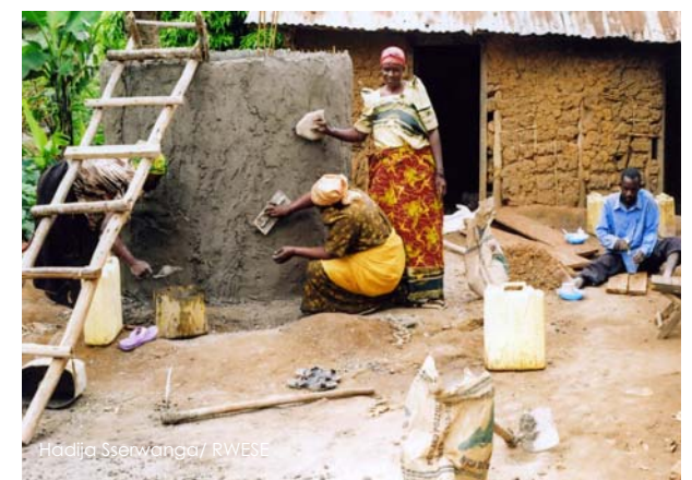
Kyotera, UGANDA. Construction of a Rain Water Harvesting Tank by women's group for an old widow. This will provide clean water close to her home.
